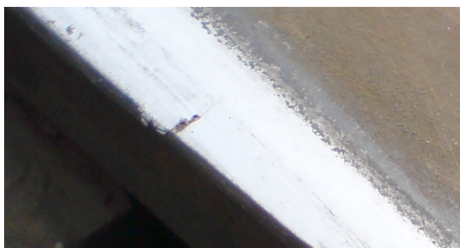
Figure 11 – VAE cross, R-65 1/11 cross-slide, Aizkraukle station
